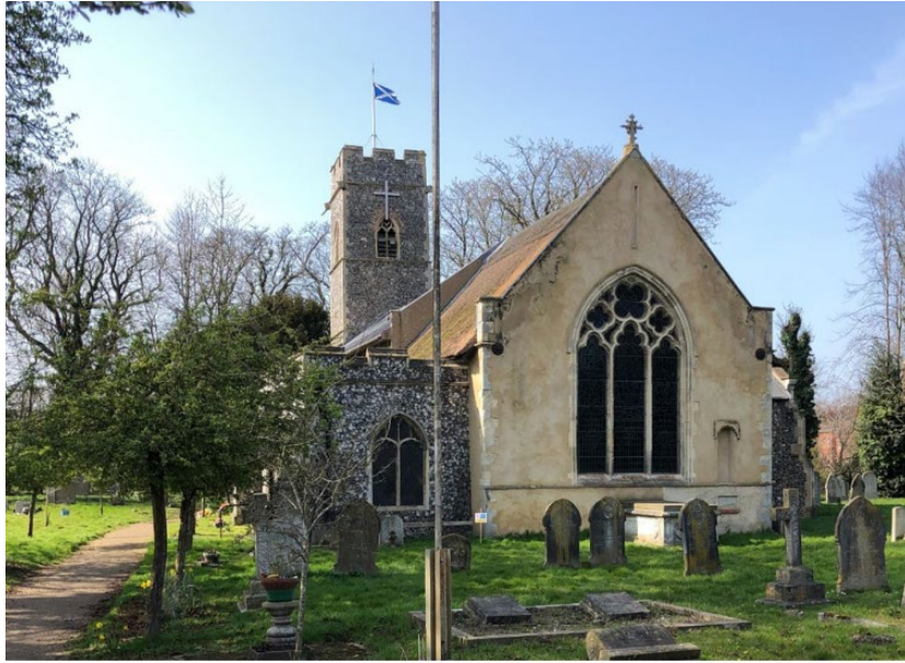
Figure 23- St Andrews Church
